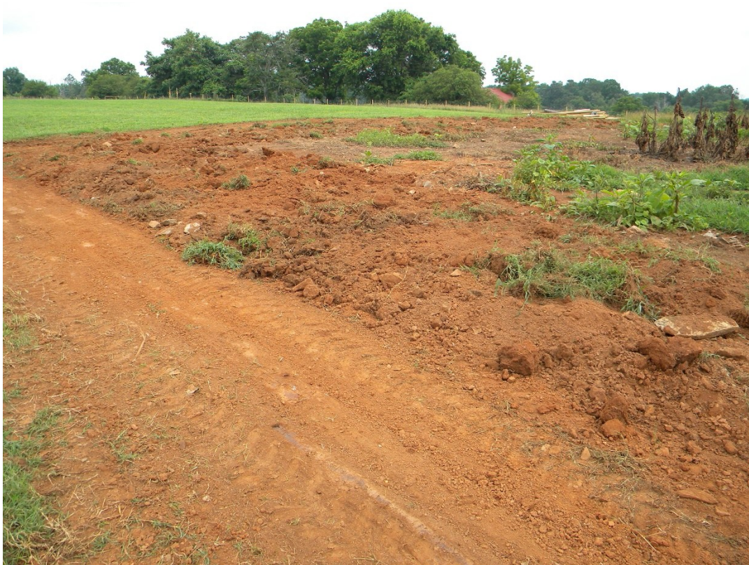
Taken 13 June 2018 by Beverly B. Wiggins showing removal of wall
